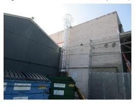
Exterior wall materials (reinforced board-form concrete; corrugated metal cladding)
