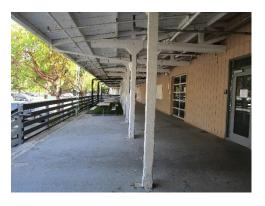
Exterior cannery features (concrete loading platforms; cooling porch at rear of building; exterior shed awnings with wood post-and-beam construction)
